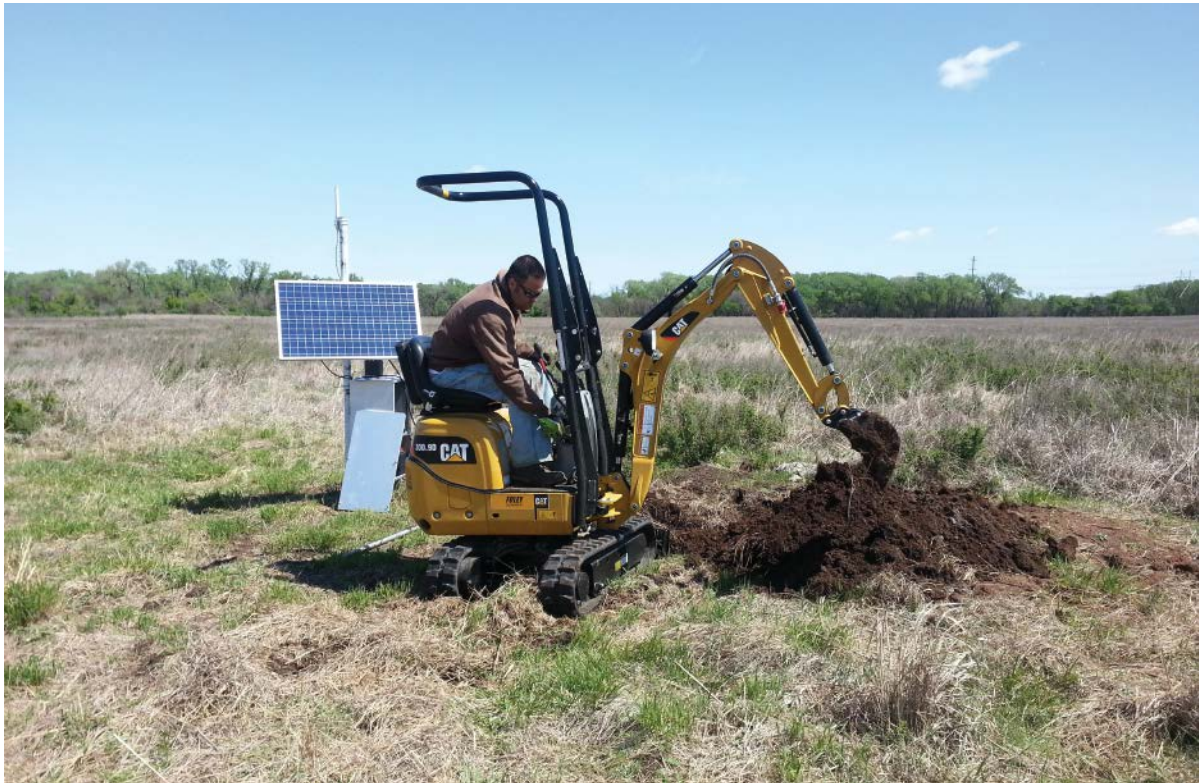
A member of the Kansas Geological Survey field crew installs a seismic station in south central Kansas. Credit: Shelby Peterie
